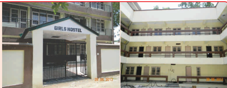
CONSTRUCTION OF GIRLS HOSTEL IN EXISTING POLYTECHNICS
